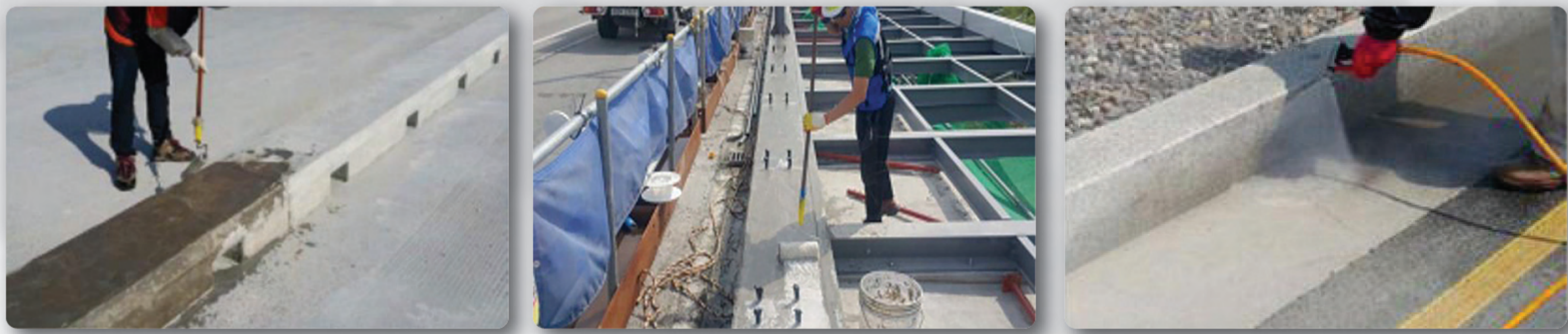
A protecting method by using hydrophobicity nano-sized inhibitors
